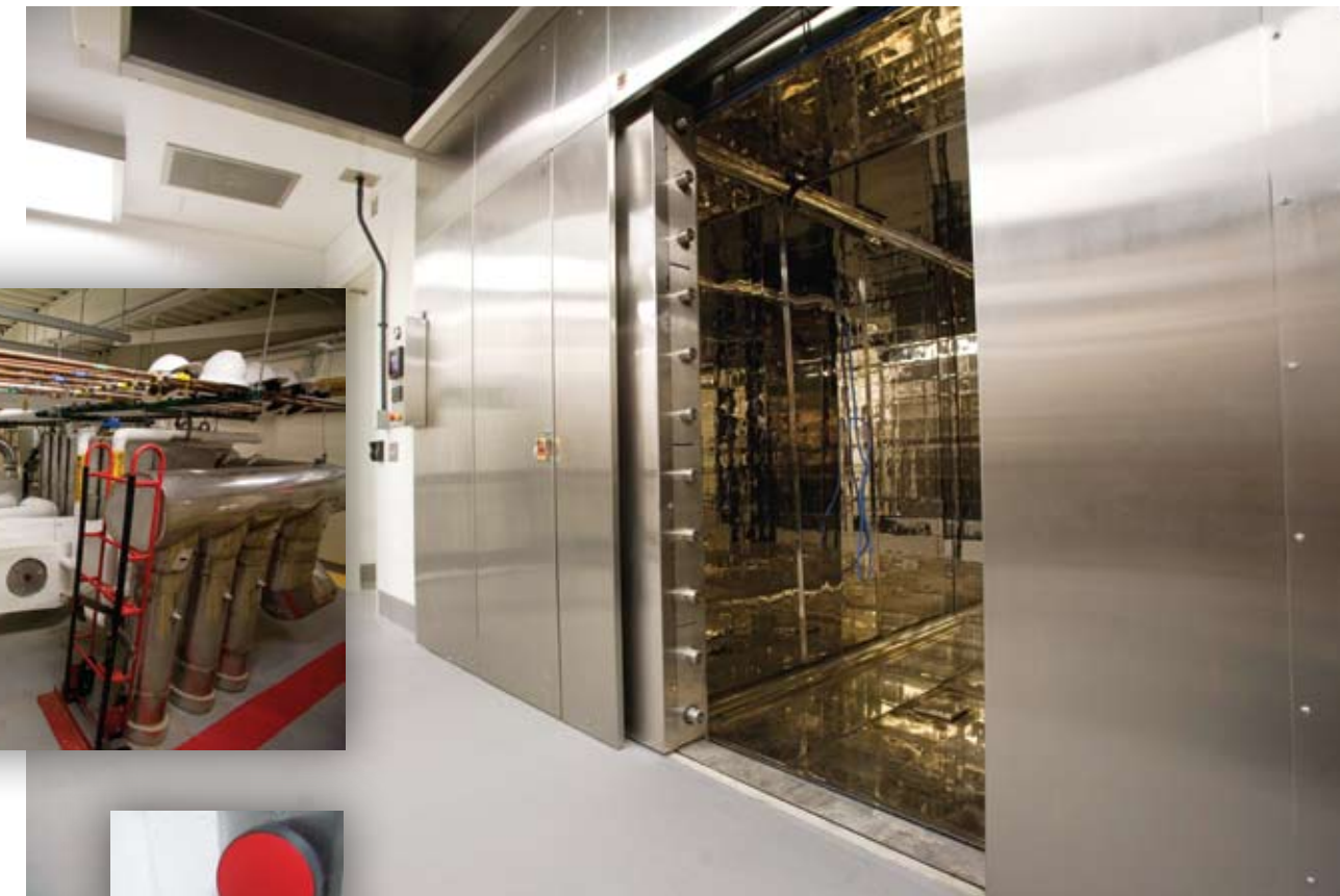
Clockwise from above: An elevator-sized autoclave at the Ricketts lab is big enough to disinfect large equipment or entire racks of contaminated cages; fingerprint scanners add extra security at lab entrances; and a sophisticated air-handling system controls and filters all airflow into, within and out of the labs. Photos by John Zich
